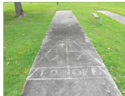
Two shuffle board courts and bench. Condition: fair-poor Needs resurfacing.
