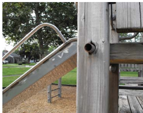
Older playgrounds rarely meet current safety inspection due to items like protrusions from the structure. Condition: poor (Remove)
