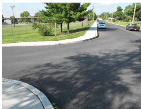
Entrances: Good visibility and site lines. 1-2 +/- year old bituminous surface Condition: Excellent
