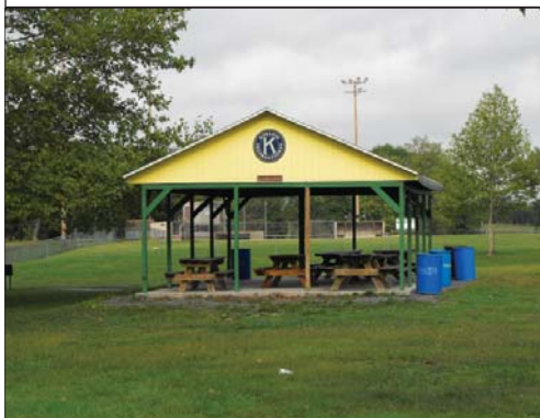
Kiwanis Shelter: Wood frame and roof with asphalt shingles Condition: very good.
