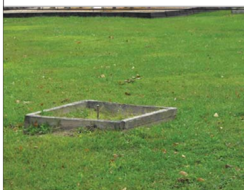
Horseshoe pits- Condition: poor. Drop the pits flush with the ground and provide sand. Provide the rod when the pavilion is rented for easier maintenance.
