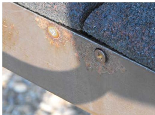
Bolts always have nuts and washers facing down. Current condition is considered a strangulation hazard
