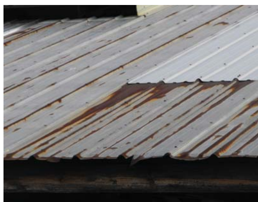
Rusting steel roof with no paint
