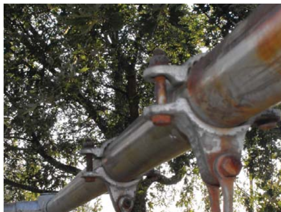
Bolts always have nuts and washers facing down. Current condition is considered a strangulation hazard
