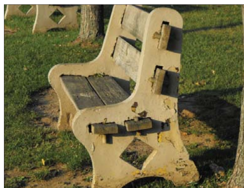
Playground benches Condition: fair-poor Replacement of wood needed on many benches. Visually the benches need scraped and painted especially on those with dedication plaques.
