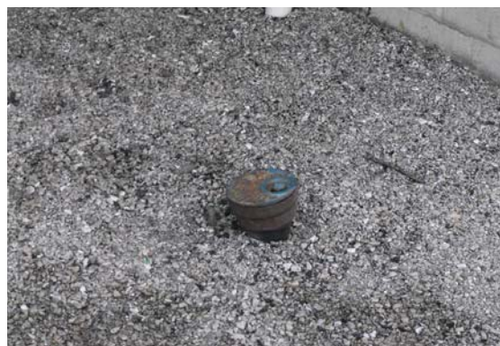
Trip hazards in bituminous such as this meter cap.
