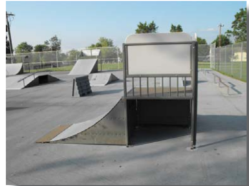
Skate piece - Condition: excellent Special tips on structures and concrete footers provide excellent foundation for a system on bituminous paving.
