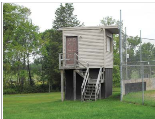
Press Box for Baseball Field Condition: fair. Stairs need rebuilt and barrier railing needs replaced ASAP.
