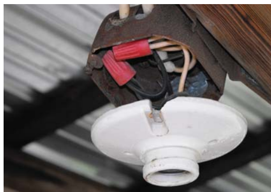
One of many exposed electrical wires. Pavilion electrical safety condition is poor.
