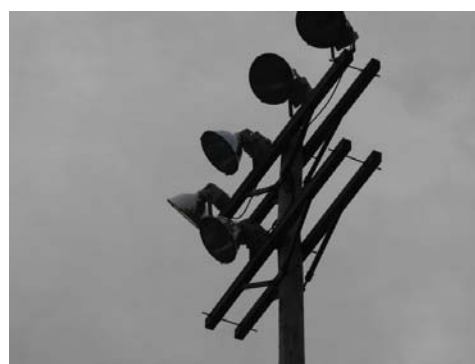
Lights are older with costly replacement bulbs and upgrades
