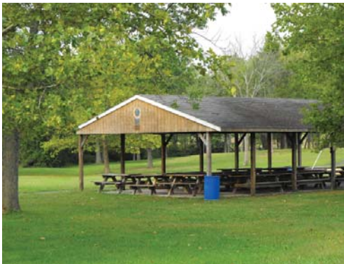
Lions Pavilion Wood frame and roof with asphalt shingles. Condition: good
