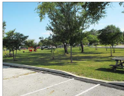
Curb tapers: Curb tapers are primarily for riding mower access over curbs. No pathway provided for ADA access to tables.
