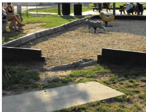
Walkways is intersected by tree root and grass. There is not ADA access to the playground.
